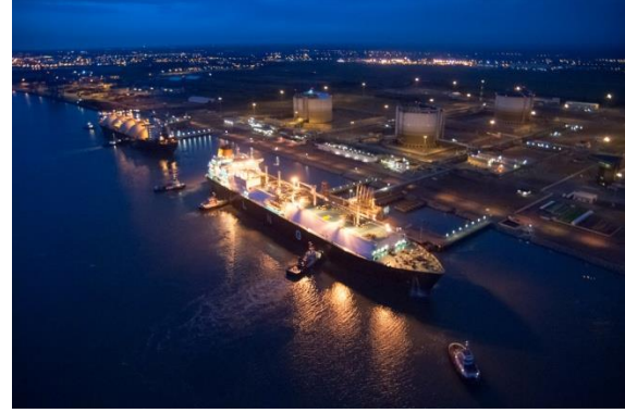
Montoir terminal, transshipment operation
